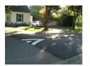
Speed Humps are designed to reduce vehicular speed on residential local or collector streets that have a single lane of travel in each direction. While generally effective in reducing vehicle speeds and
